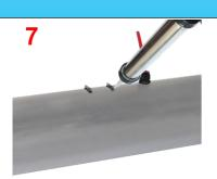
7: Seal the clearance between the metal tabs and the outer sheath of the piping with a silicone or elastomeric sealing resin. Wrap the mechanical protection around the insulation, making two straight cuts for the legs
