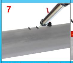
7: Seal the clearance between the metal tabs and the outer sheath of the piping with a silicone or elastomeric sealing resin. Wrap the mechanical protection around the insulation, making two straight cuts for the legs
